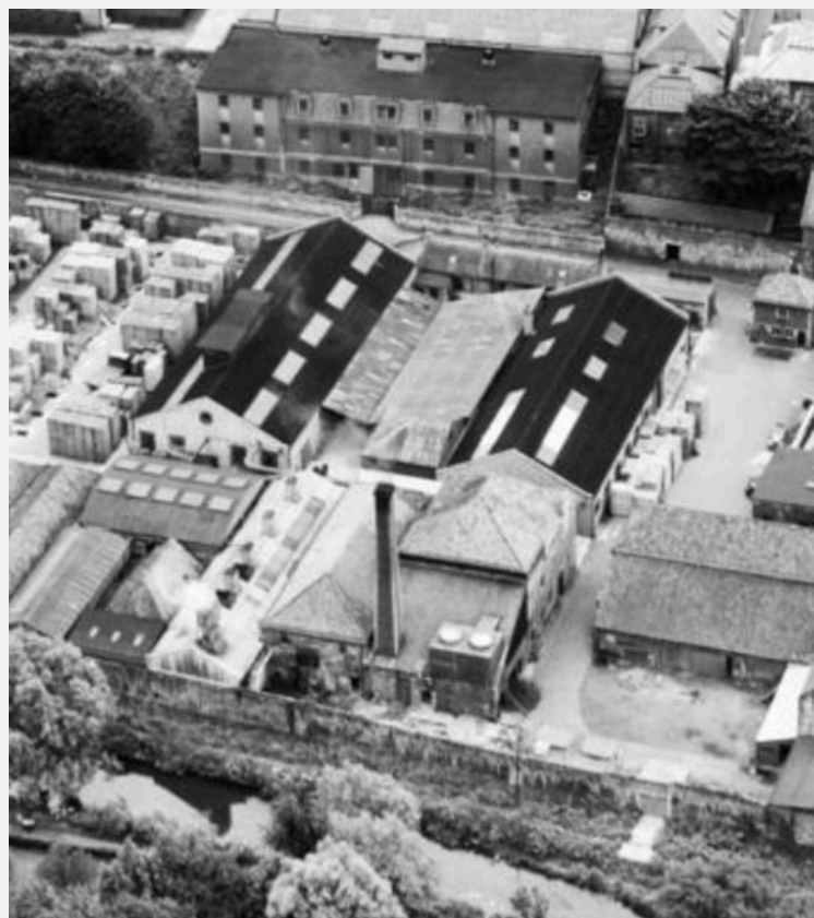
aerial photograph taken facing south of the distillery in 1949.
